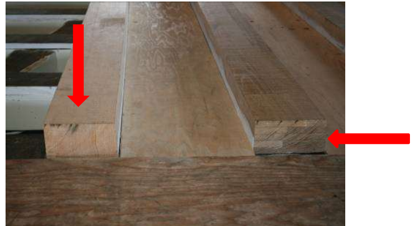
Solid fir decking (left) & laminated white oak (right)
