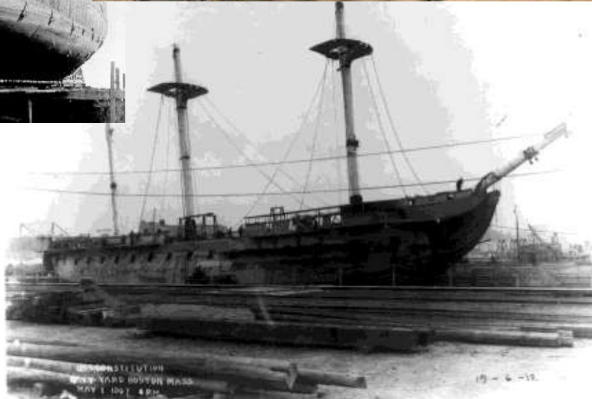
1906-07 re-building,; open waist re-created, using 1812 USSC model
