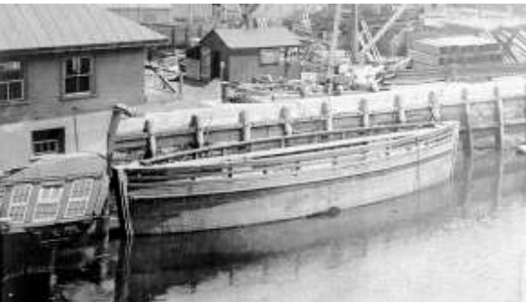
Original 1833 wooden caisson, photographed in 1903. (BNHP photo)
