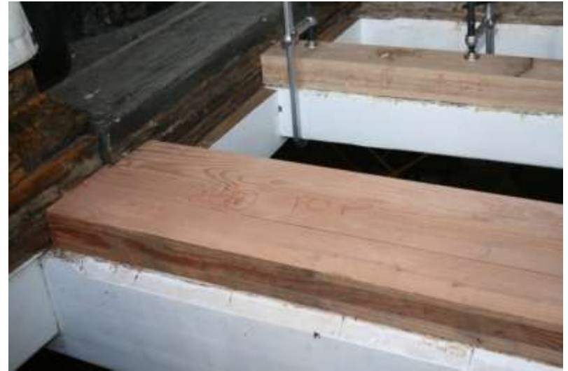
Camber re-created by installing shims on each deck beam & ledge (above)
