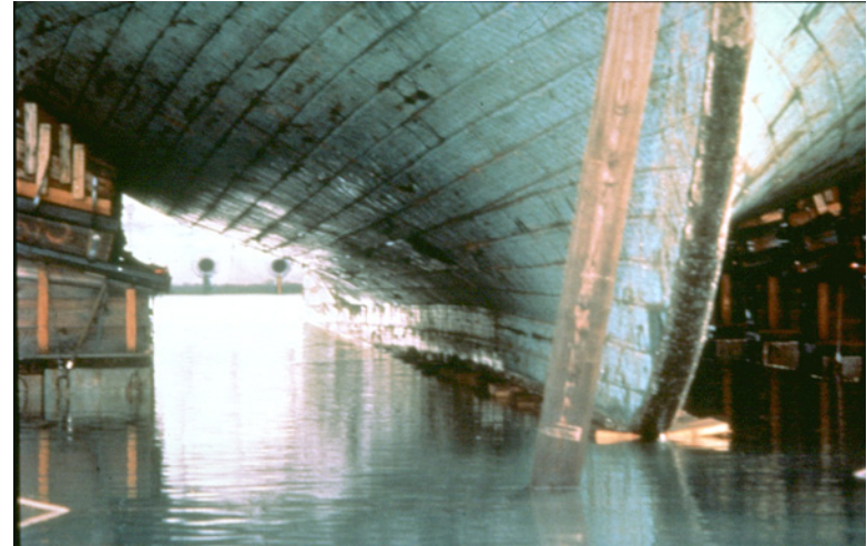
Detail of copper cladding on USS Constitution in drydock, ca. 1995
