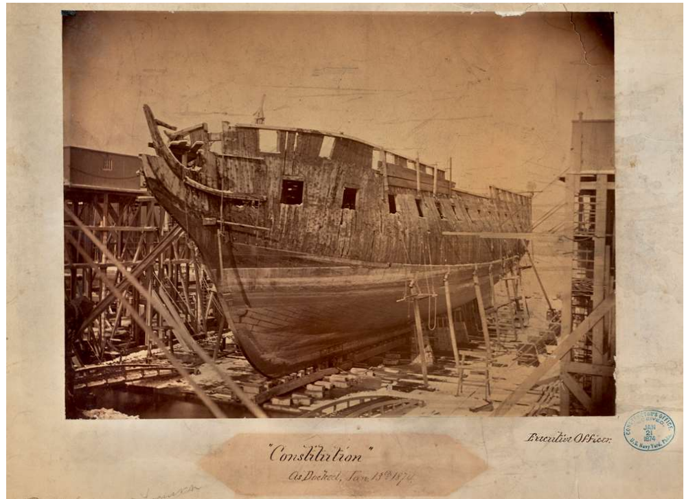
Figure 7: “Constitution as docked, Jan. 13, 1874.” This photograph shows the ship hauled from the water and stripped of its planking during the 1874 restoration in Philadelphia. USS Constitution Museum Collection, 1528.1.
