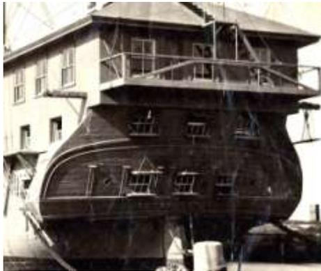
c.1897 photo, USS *Constitution* at the Portsmouth Navy Yard. Note the lack of detailed decoration on the ship's stern; portholes have replaced the 2 outboard-most windows and only molding, pilasters flanking the windows & ports, and the ship's name relieve the starkness of the large, flat ship's stern. US Navy Photo.
